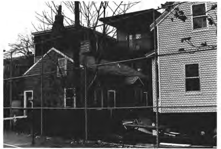
72 Dane Street, ca. 1750. Near the route of Washington Street, this three bay house is situated near the intersection where the first resident of Charlestown "beyond the Neck" settled.
