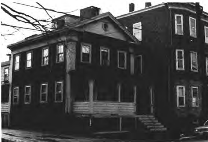
384 Washington Street, ca. 1855. Washington Street near the Cambridge line (and Kirkland Street) was once a corridor of fine homes on spacious lots. This house, owned by jeweler Charles Schuebeler in 1869, has an array of intact original details which surround the twentieth century asphalt siding. Of particular significance is the central oculus surrounded by a carved wooden garland.
