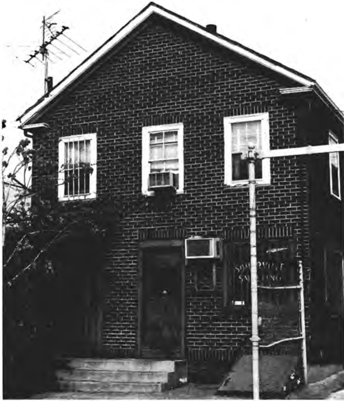
14 Joy Street, ca. 1855. Joy was one of the first streets platted in the real estate development which occurred around the Asylum grounds and railyards shortly before the Civil War. Although many streets were platted, only a few were ever developed. By 1890, Joy, Linwood, Chestnut, Poplar, London and Fitchburg Streets were filled with closely-built houses and numerous rowhouses intended for laborers. When the area was cleared for an industrial park in the 1950s, this was one of the only houses left standing. This house gives an indication of the appearance of other houses in the area, with a standard plan of 3 bays and a sidelit side entry (with an interesting entrance decorated with punched foliate panels and pendant brackets).
