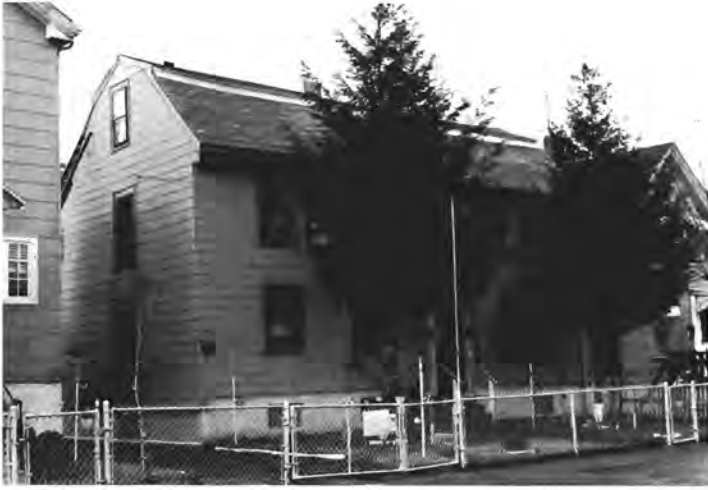
6 Kent Court, ca. 1750. This five-bay, gambrel-roofed Colonial house was moved to its current location from Somerville Avenue. Nearby, Kent Street was an early connector between Beacon Street (1813) and Milk Row. After the Civil War, Kent Court was squeezed between the Reitenbach Brothers Mink Tannery, the Middlesex Bleachery, and the tracks of the Fitchburg Railroad.
